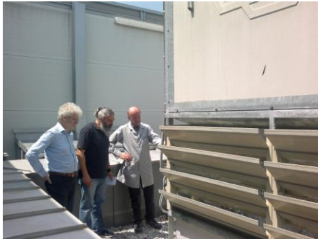
Figure 12: Inspection of the evaporation towers at the rooftop.
