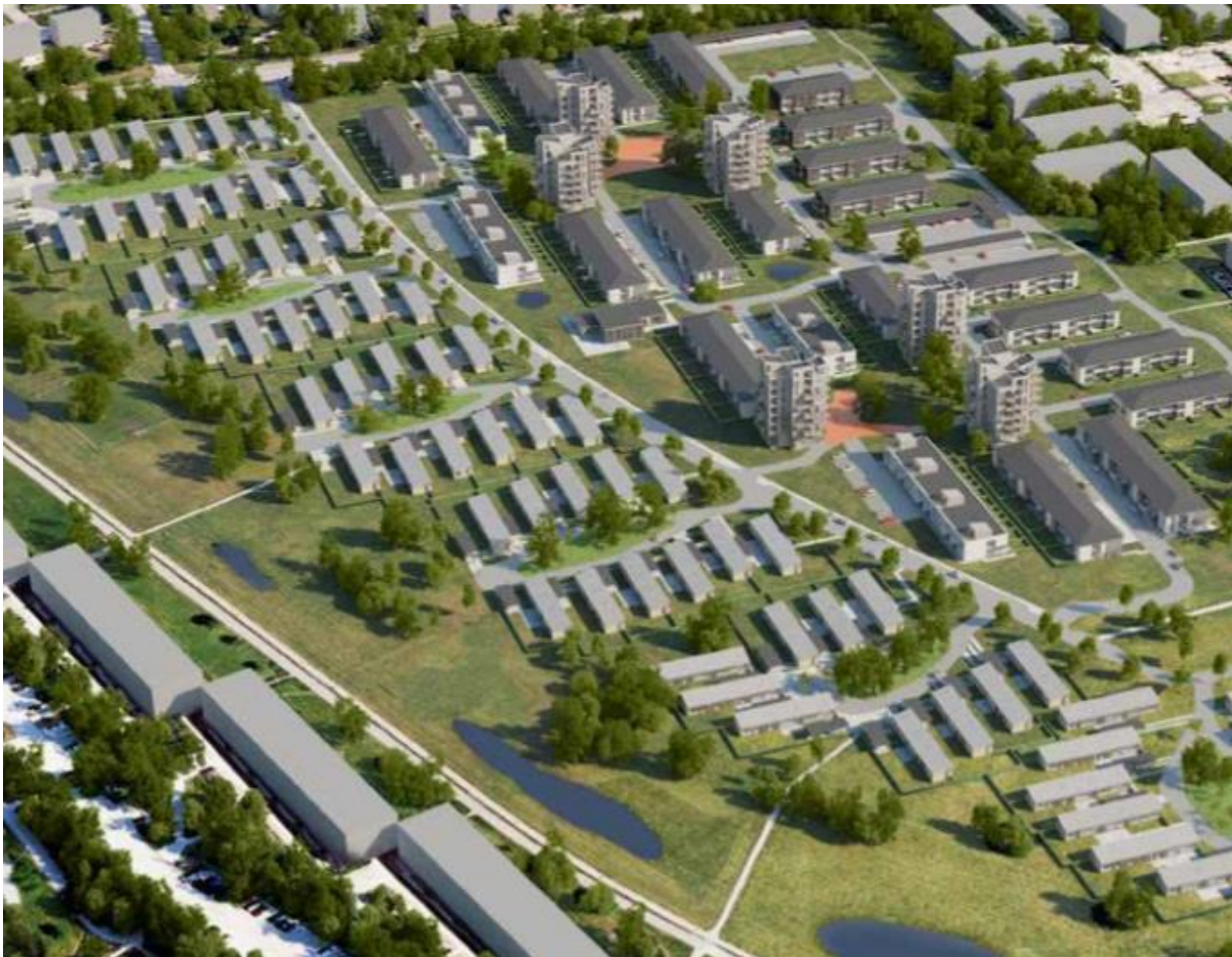
Figure 1 Kildeparken housing area, Aalborg, Denmark
